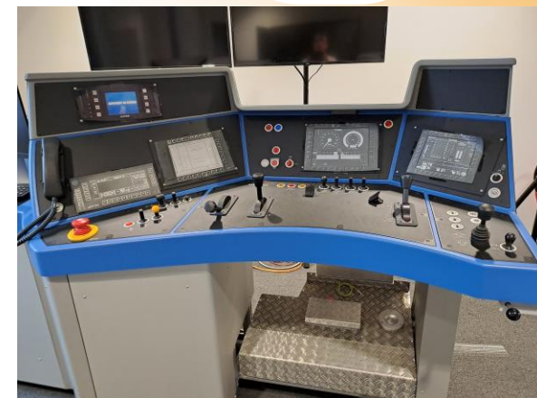
Connexion with DB Cargo equipments
