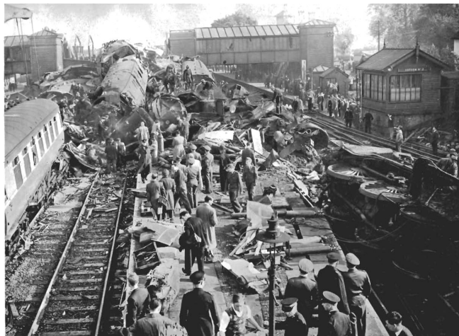
Figure 3.1: Double collision which occurred on 8th October 1952 at Harrow and Wealdstone Station
